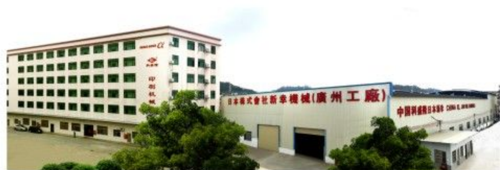
Guangzhou Shinko Plant
